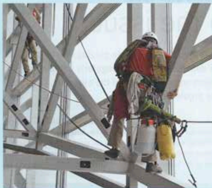
Climbing in the structural frame to the rappelling point.
